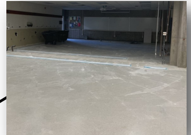
Swing Space - Fine Arts (Old SEM) [Construction]
