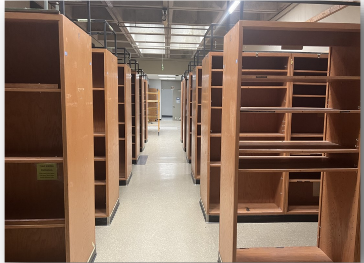
Swing Space—Fine Arts—Demolition in Progress
