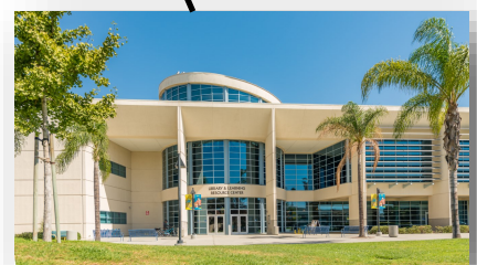
LLRC Secondary Data Center (Phase II) [ Implementation ]
