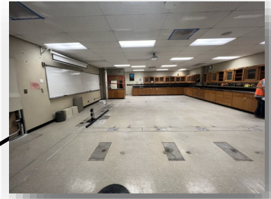
Swing Space - Fine Arts (Old SEM) [Construction]
