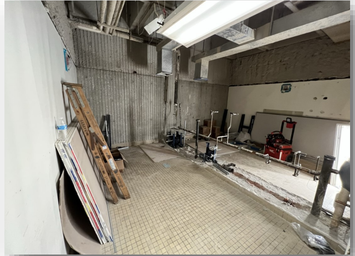
Swing Space—Fine Arts—Demolition in Progress
