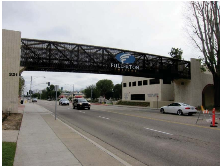
Figure 27. Pedestrian Bridge and Student Center constructed in 1984
