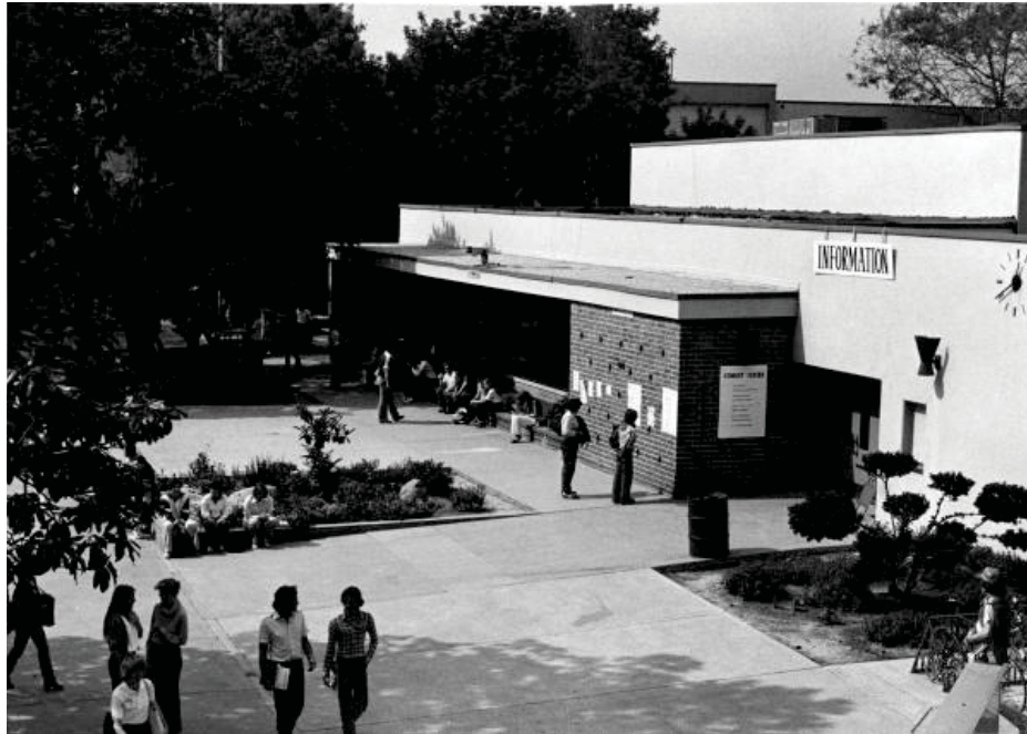
Figure 18. Student Center constructed in 1957 and demolished in 2007
