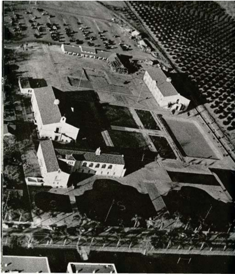
Figure 7. Aerial photograph from 1940 showing the FJC Campus and Vaughn's many accomplishments during his time with FJC (Richey et al. 2012)
