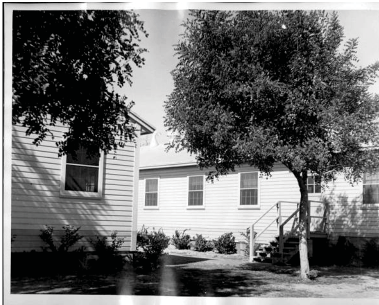
Figure 14. T Shacks used for classroom spaces starting in 1946
