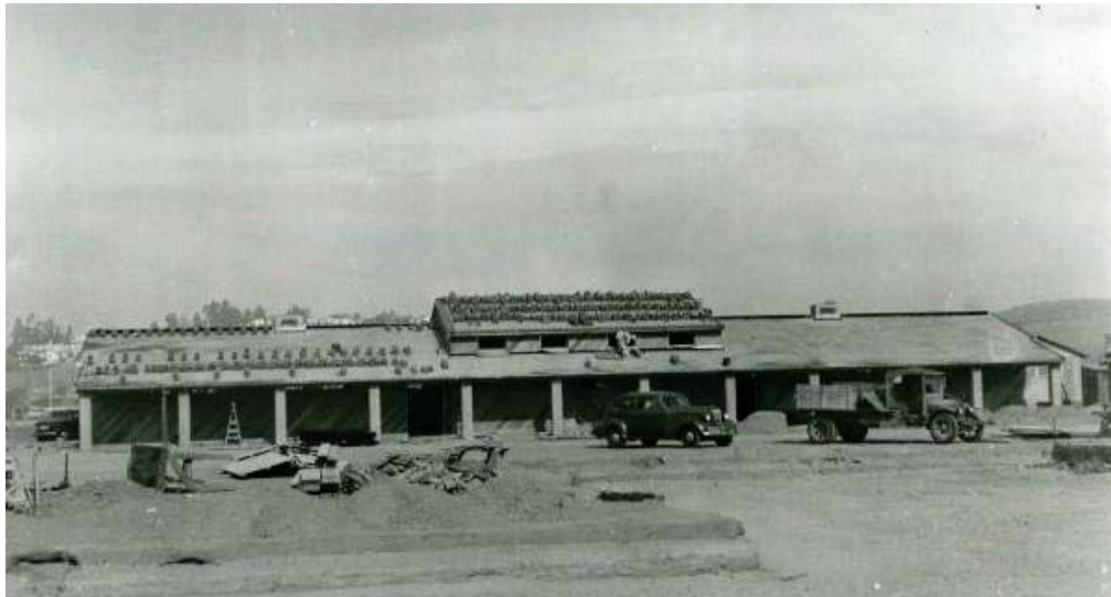
Figure 12. Student Union building under construction in 1939
