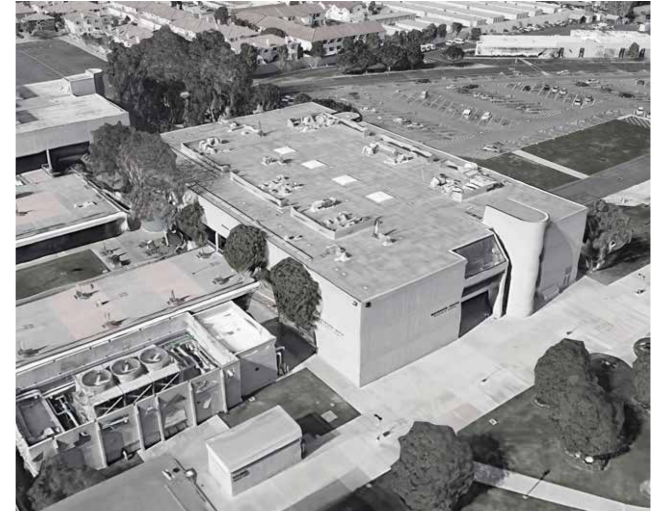
EXISTING SEM BUILDING SOUTH WEST CORNER
