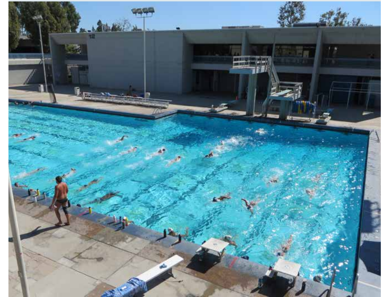
EXISTING SWIMMING POOL
