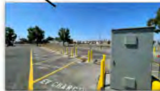
Electrical Vehicles (EV) SCE Charging Stations-Lot 4 [Construction]
